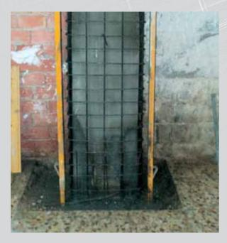
Prior reinforcement and screed of columns with MORCEMREST EF 50 in Elche (Alicante)
