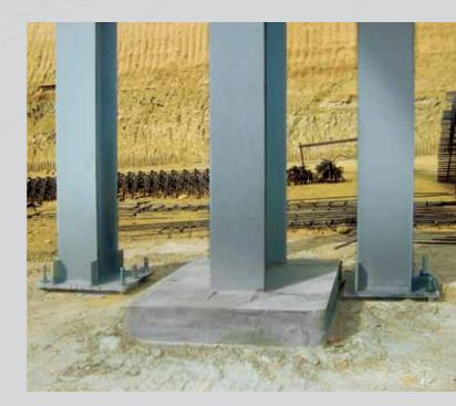
Detail of levelling and filling under anchoring plates of metal structure
