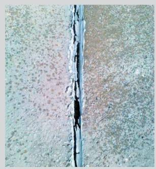
Close up of joint on water tank cover whose sealing has deteriorated over time.
