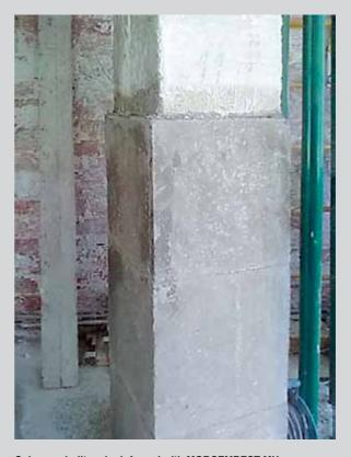
Column rebuilt and reinforced with MORCEMREST MH applied by pouring, in Tavernes de Valldigna (Valencia)
