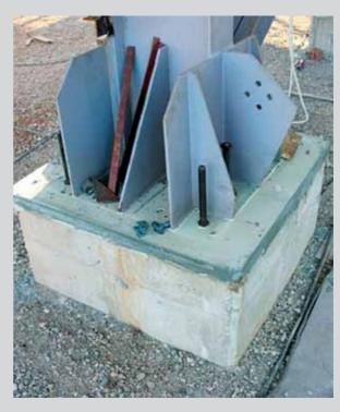
Levelling Biodiesel plant with MORCEM GROUT 500 Andujar (Jaén)
