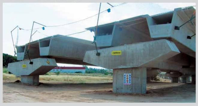
Detail of neoprene supports levelled with MORCEM GROUT 500 on the MU-31 (Murcia)
