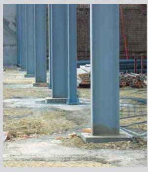
Detail of levelling and filling under anchoring plates of metal structure
